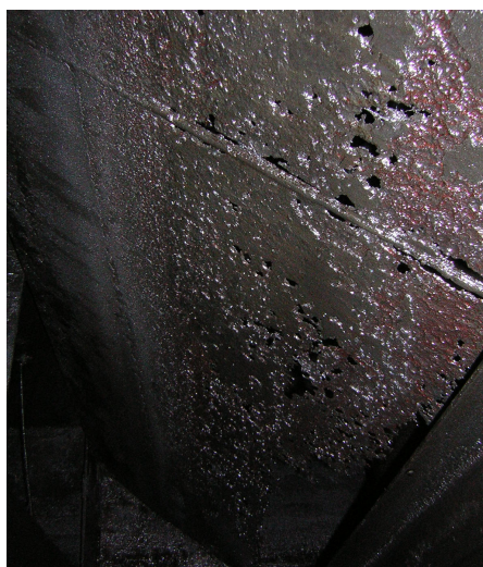
Figure 4- Photograph the zone attacked by pitting can be observed.
