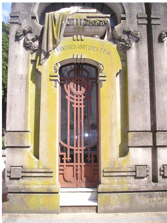
Fig. 1. Portico of the crypt of Francisco Arrechea (crypt F87), which is of architectural interest because of its Art Nouveau style. The yellowish coloration is indicative of the presence of Caloplaca austrocintra .
