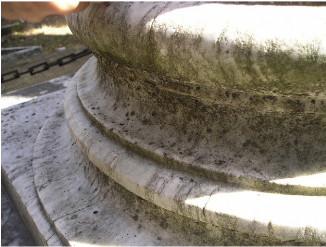
Fig. 2. Biofilm on the marble column of crypt C95.
